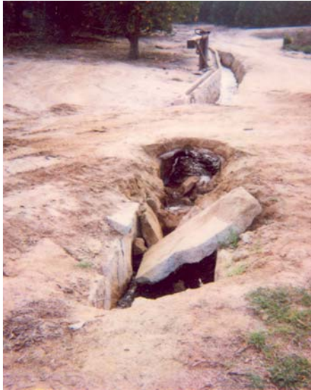
Collapsed flume east of Red Hill, photo taken in 1993.
